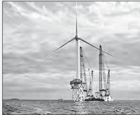
Wind Turbine Installation
