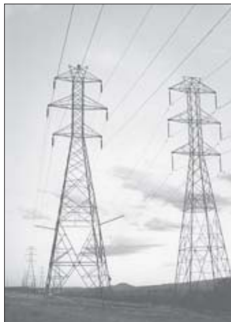
Do we really need more transmission lines marching across the hills of what few green spaces are left?
