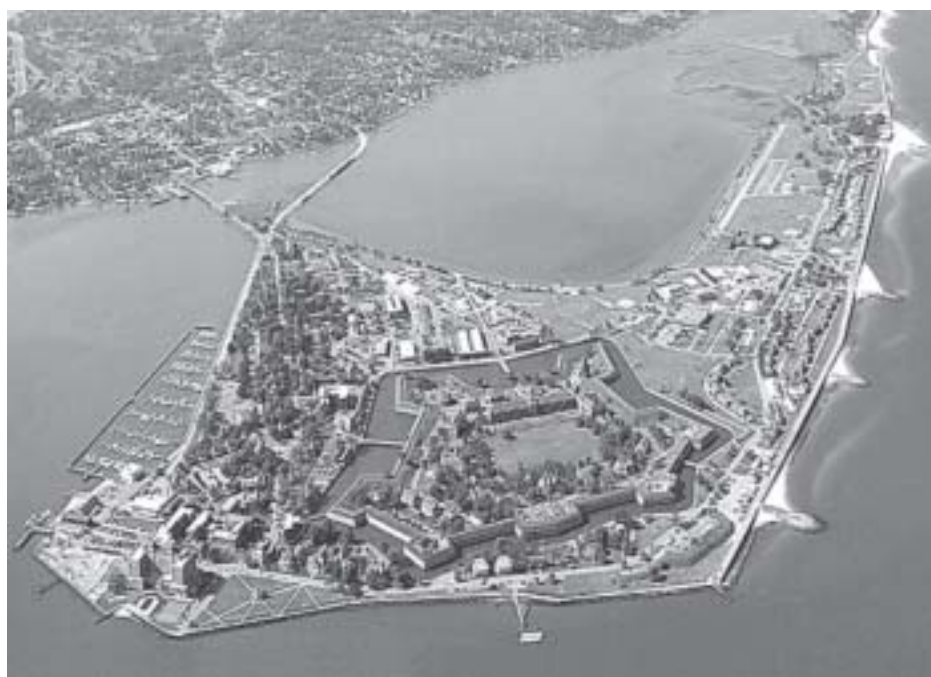
Aerial view of Fort Monroe at the mouth of the Chesapeake Bay
